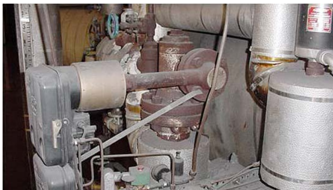
Modernizing feedwater heater level controls allows operators to better manage controllable losses while significantly reducing maintenance costs. Torque tube displacers (above) are common in the industry and one of the easiest to retrofit.
