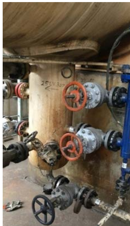
Figure 9: Boot for separation in a refinery (GWR transmitter installed in blue chamber at right)
